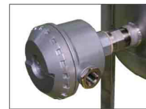
Lower level alarm for hardener tank
